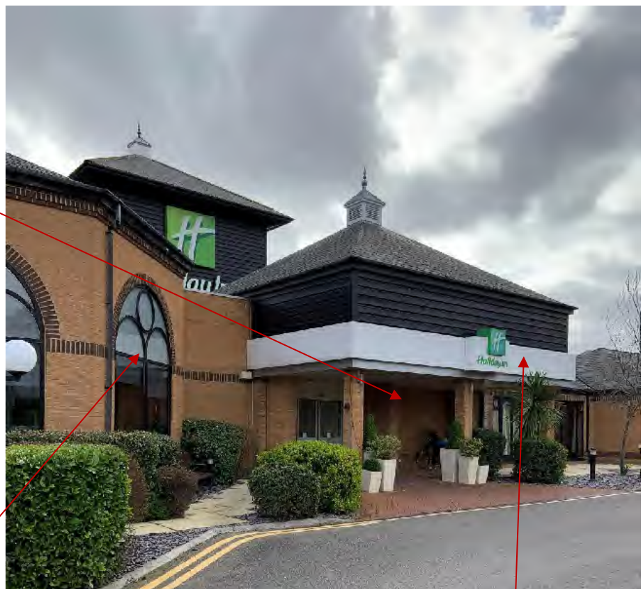
Remove cladding & replace with dark grey aluminium cladding
