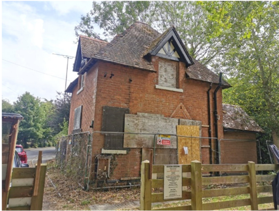
Photograph 1. View of the north-west corner of the Lodge.
