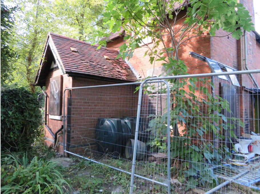
Plate 13 – General view of lodge.
