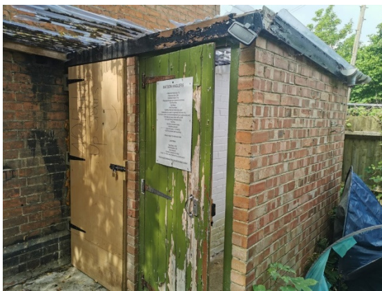
Photograph 3. View of the toilet block extension.
