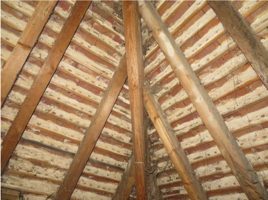
Plate 19 – General view of lodge roof.
