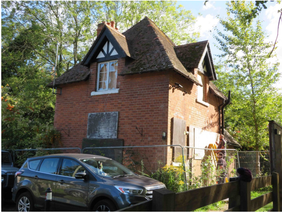
Plate 14 – General view of lodge.
