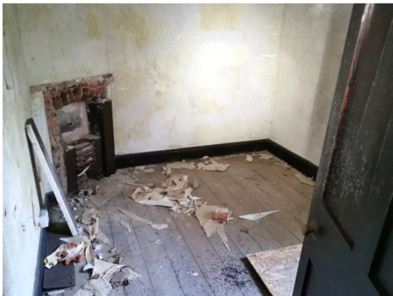
Photograph 5. View of rear upstairs room.
