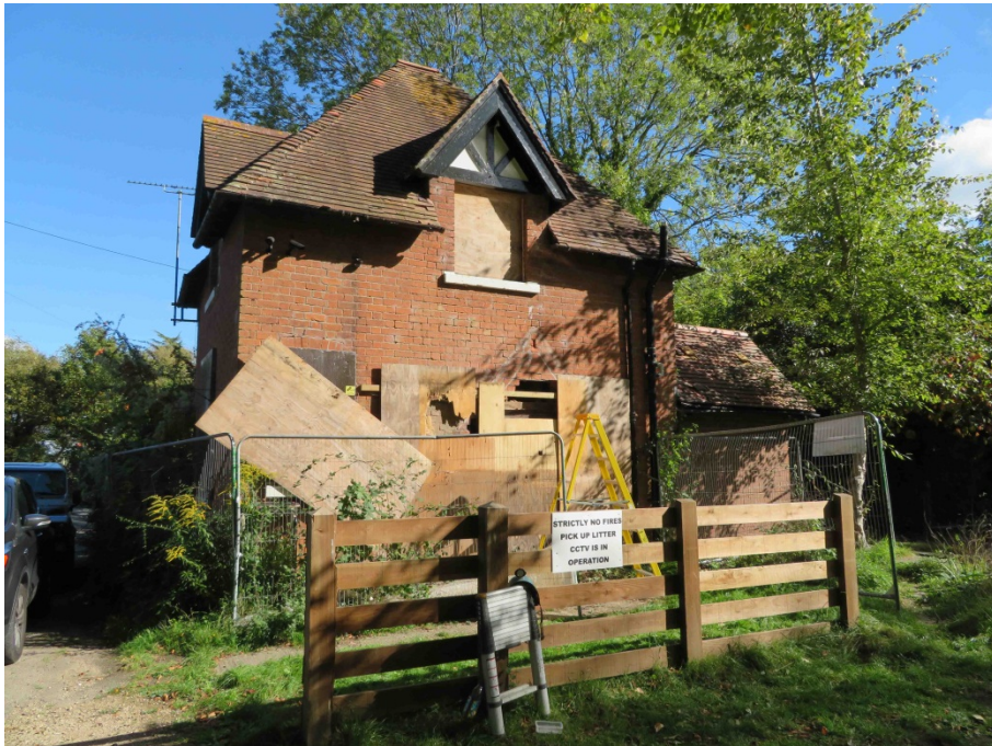
Plate 2 – Lodge Building (TN2).
