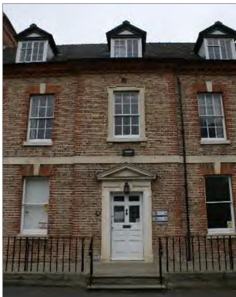
Plate 4. Fenestration pattern to ground and first floors.
