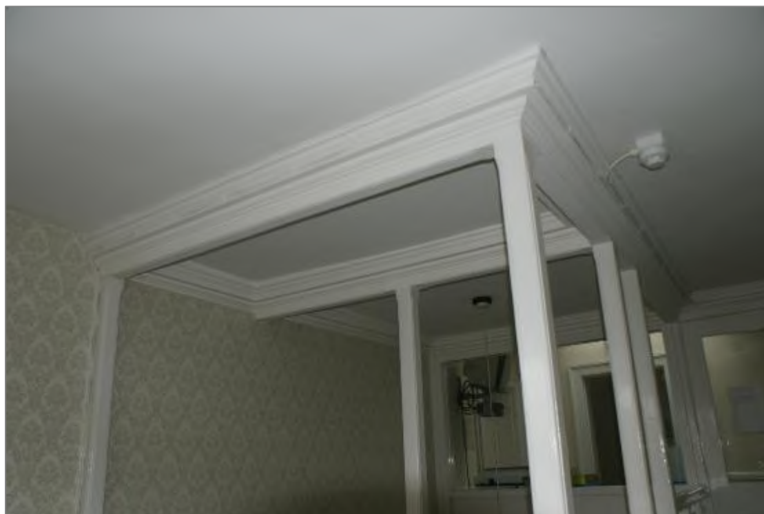
Plate 16. First floor fire lobby to principal stair.
