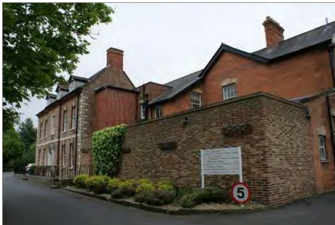
Plate 21. Piecemeal extensions relate poorly to the host building.
