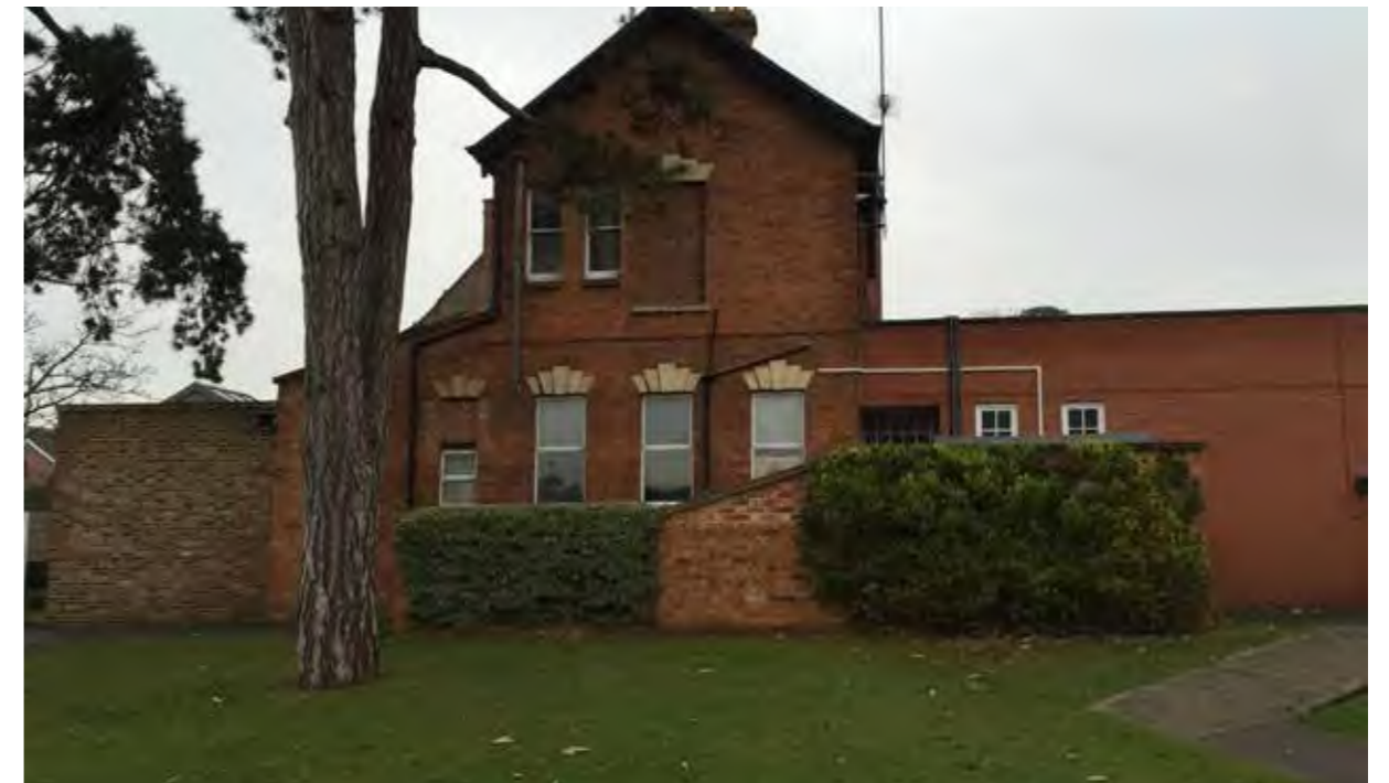
Later extension at the rear of the Manor House
