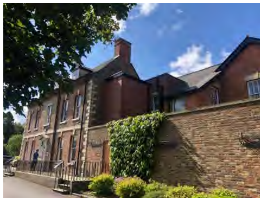
Front entrance view of modern lift shaft and single storey extension
