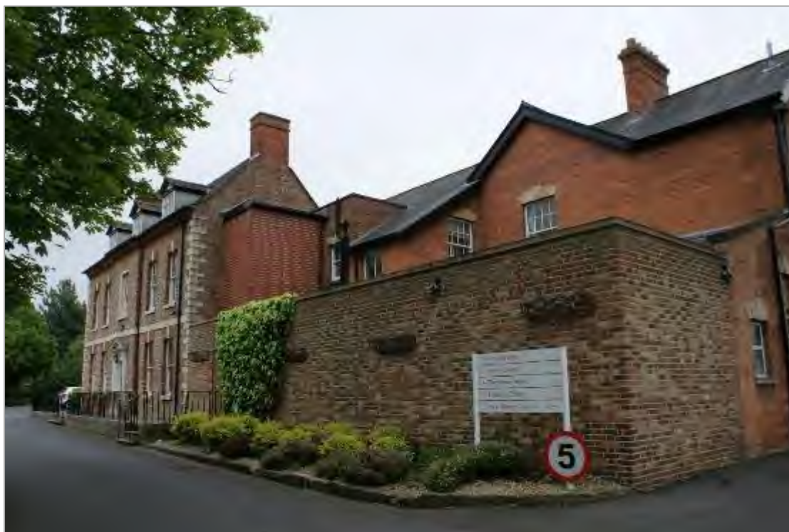
Plate 3. Late twentieth century flat roofed addition with lift shaft behind.
