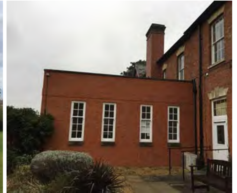
Rear modern single storey extension
