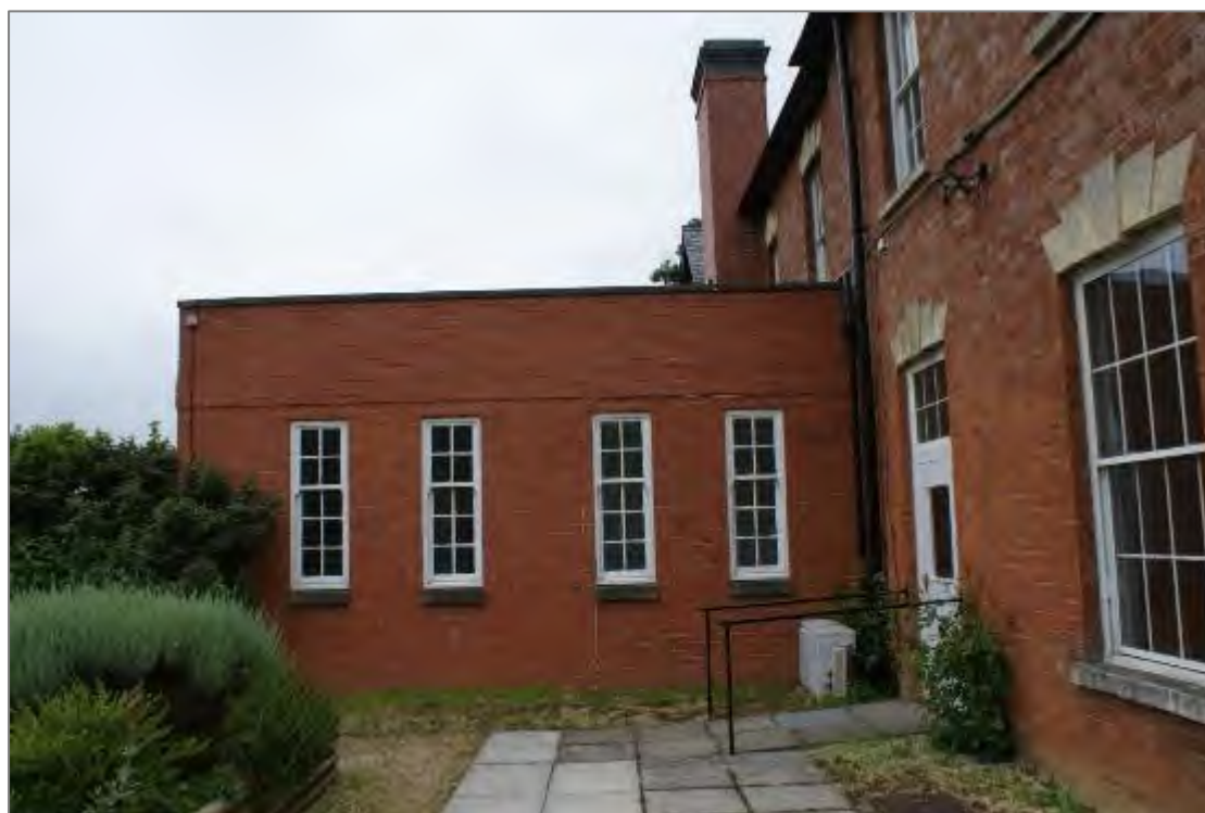
Plate 6. Windows to the east elevation of the 1981 extension.
