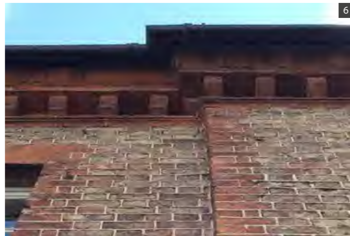
Existing brick cornice detail at the eaves of the Manor House
