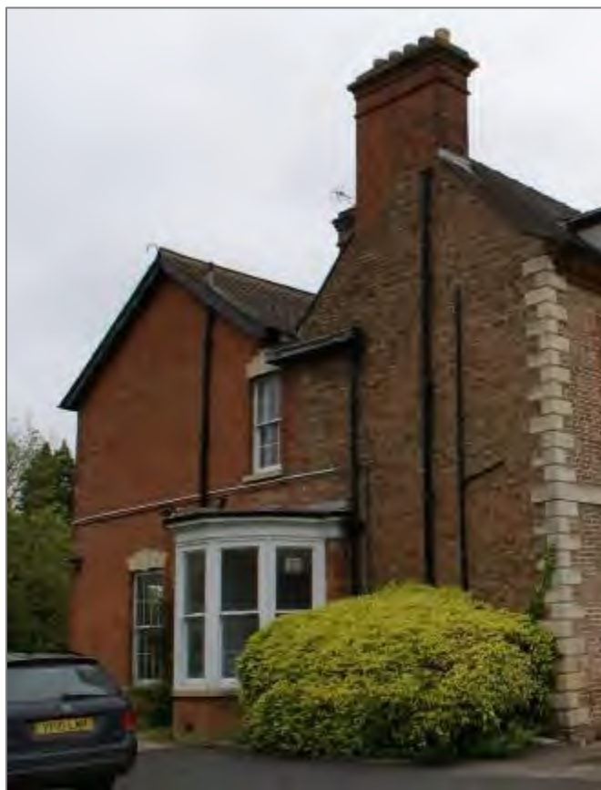
Plate 7. Bay window to east elevation.
