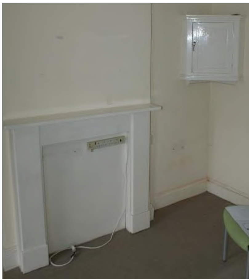
Plate 11. C19 fire surround and corner cupboard to the first floor
