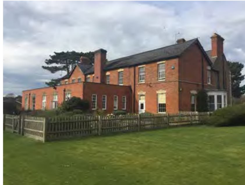
Rear modern single storey extension onto garden
