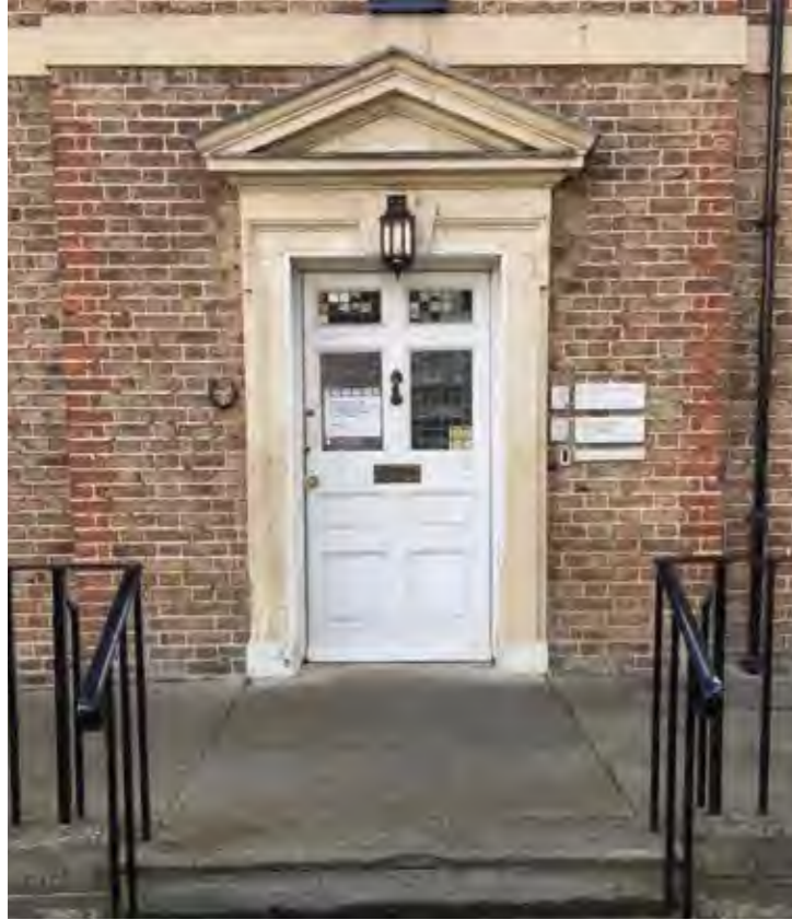
Manor House. Intricate stone detailing around the front door
