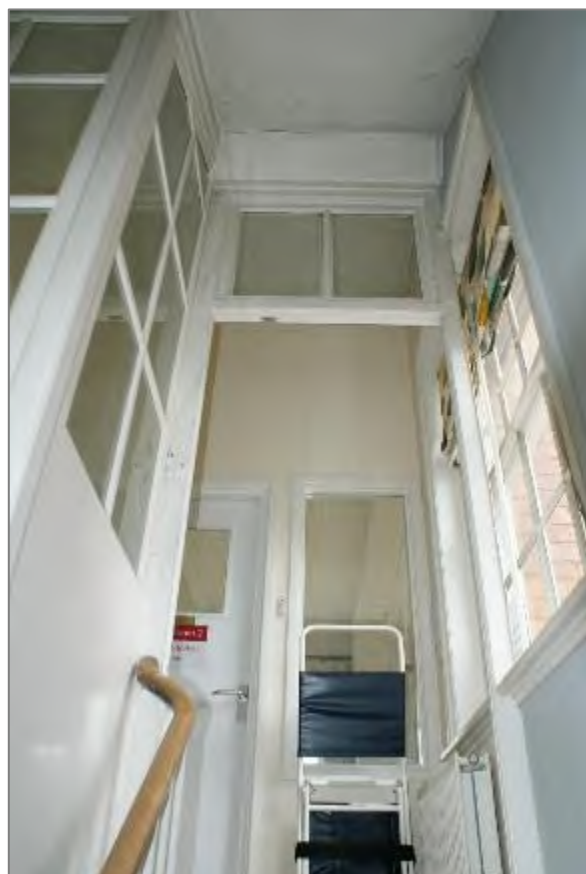
Plate 17. Fire lobby to first floor of service stair.
