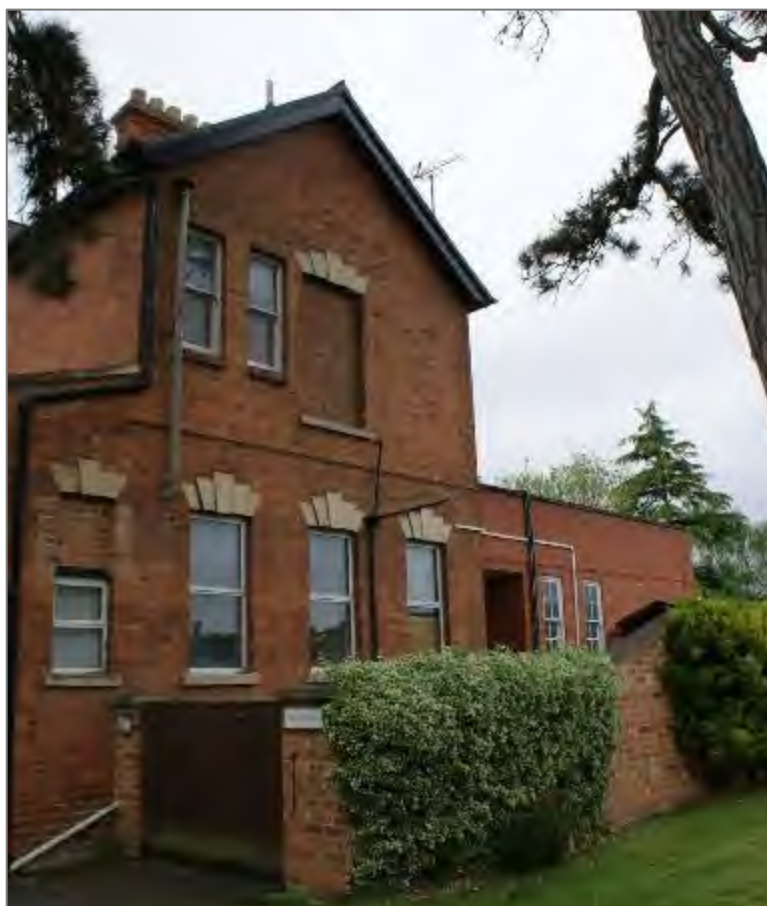
Plate 5. Windows to the west elevation.
