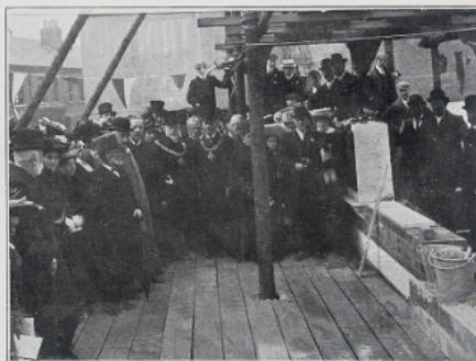
LAYING FOUNDATION STONE Photo by Fletcher, Glendon.
