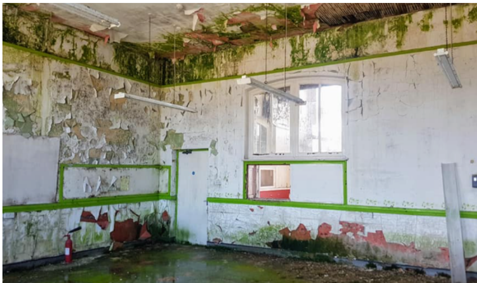
Photographs showing interior condition of the building, taken March 2020
