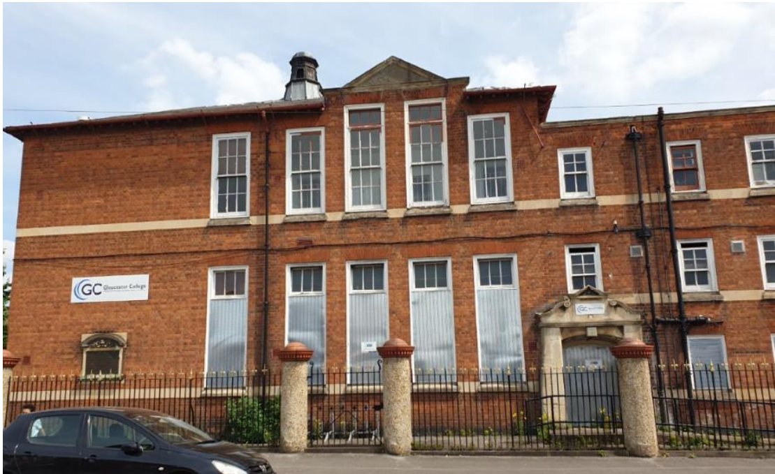
West facing elevation fronting Derby Road
