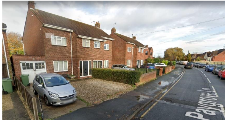
Existing housing on Paygrove Lane
