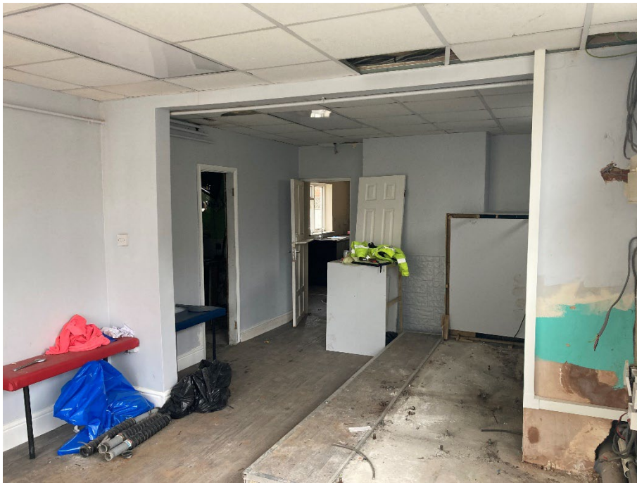
9 Interior – concrete plinths for removed washing machines
