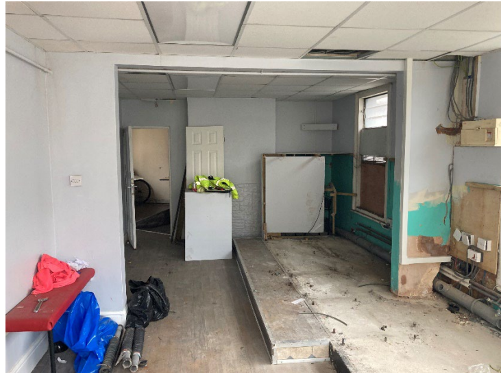
8 Interior – concrete plinths for removed washing machines
