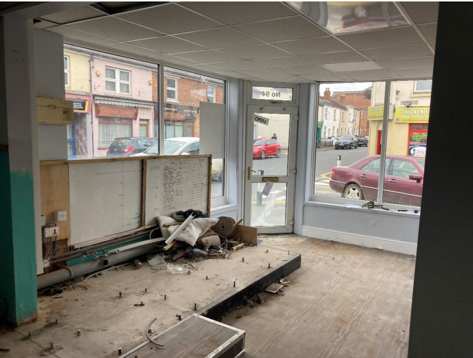
7 Interior – concrete plinths for removed washing machines
