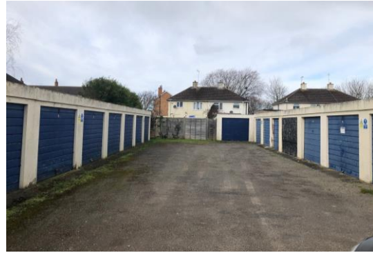
Garage structures within the application site
