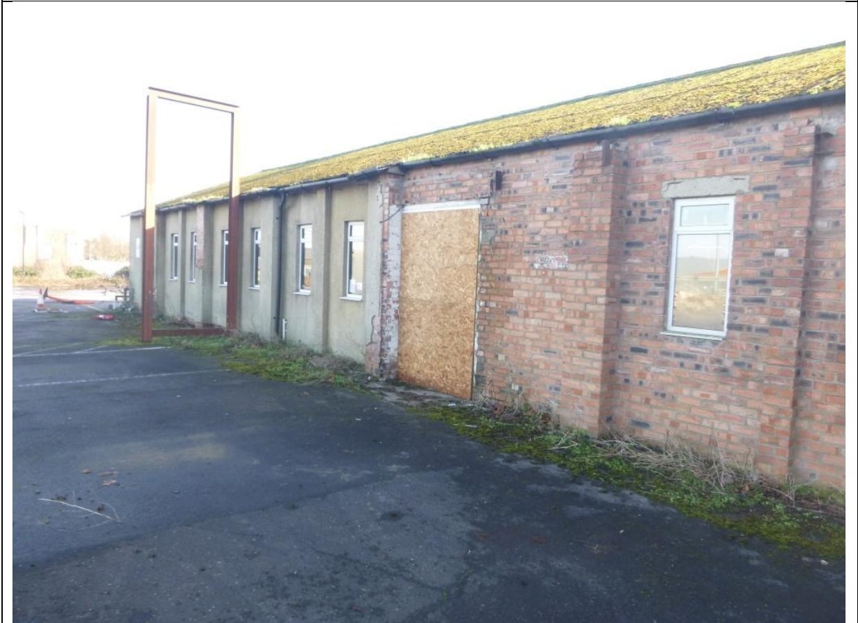
2. Former Fork Lift Repair Building
