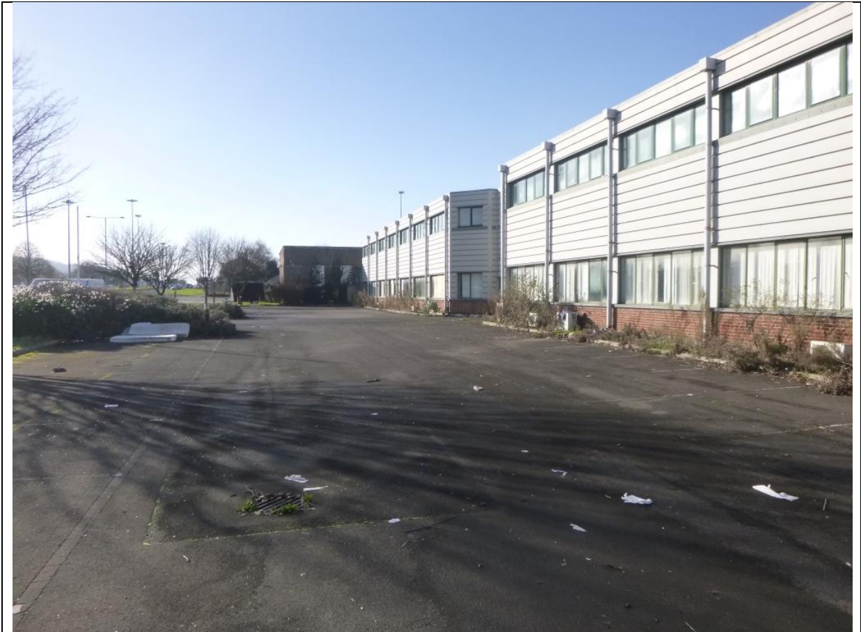
1. Car Parking east of offices
