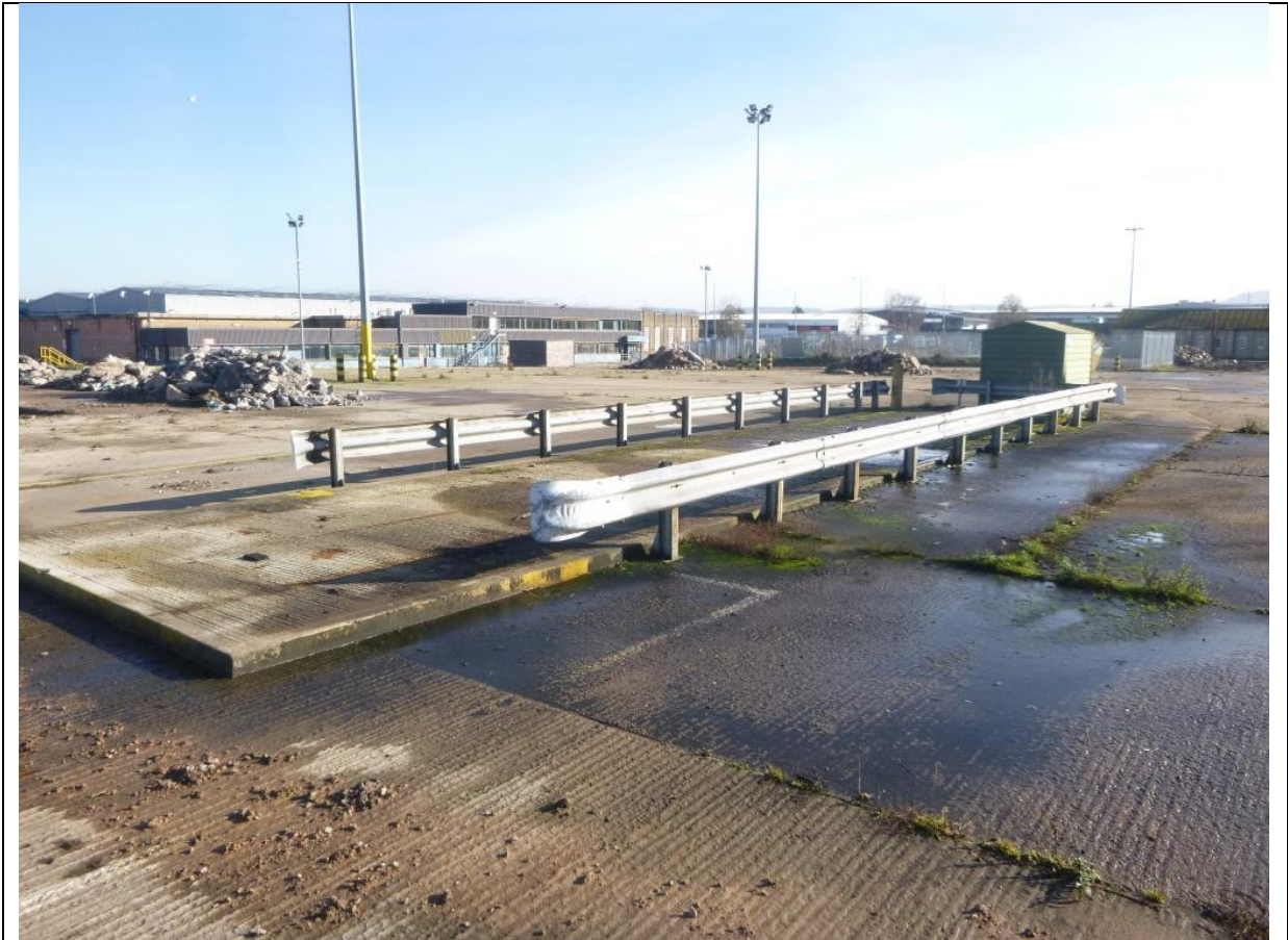
3. Former diesel AST
