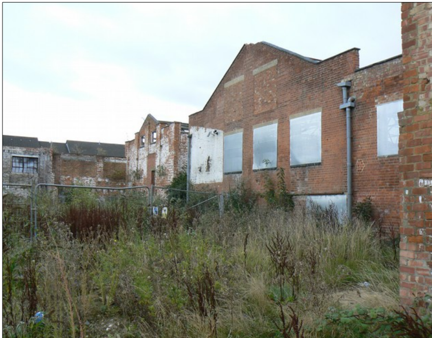
Plate 3: Southern elevations of southern range of buildings. View - SE
