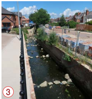
3 View from Hatherley Road.
