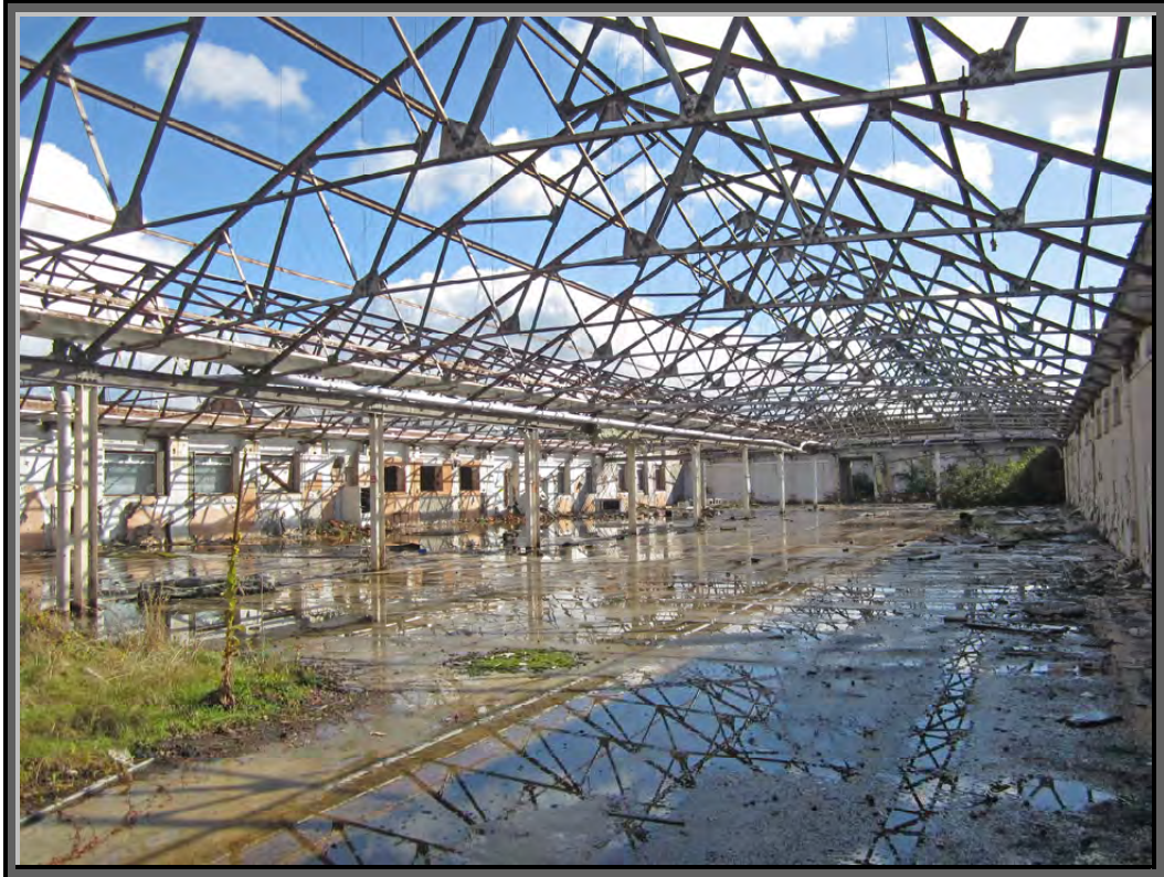
Photograph P5: showing Building 5 interior
