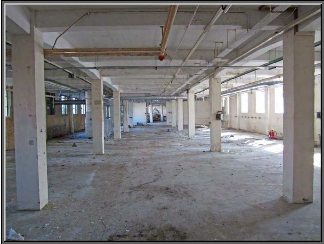
Photograph P3: showing Building 2 interior
