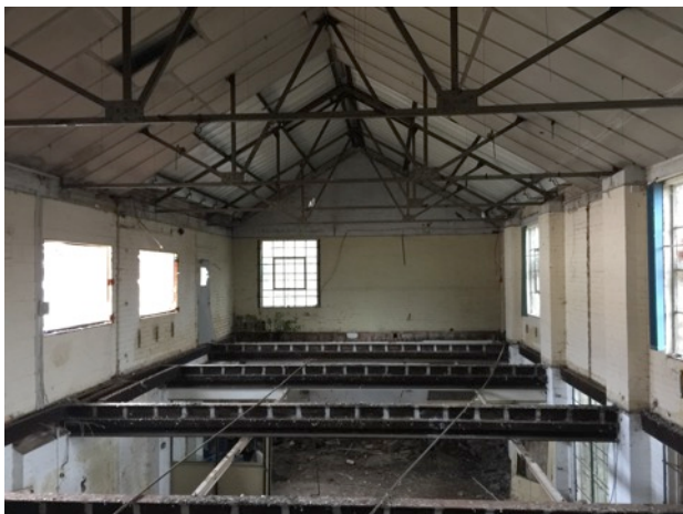
Photograph 9: Small roofed section of Building 1.
