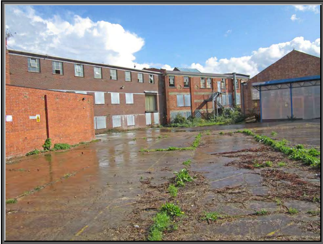
Photograph P1: showing view across main yard
