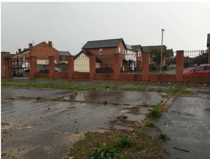
Photograph 7: Perimeter walls and railings.
