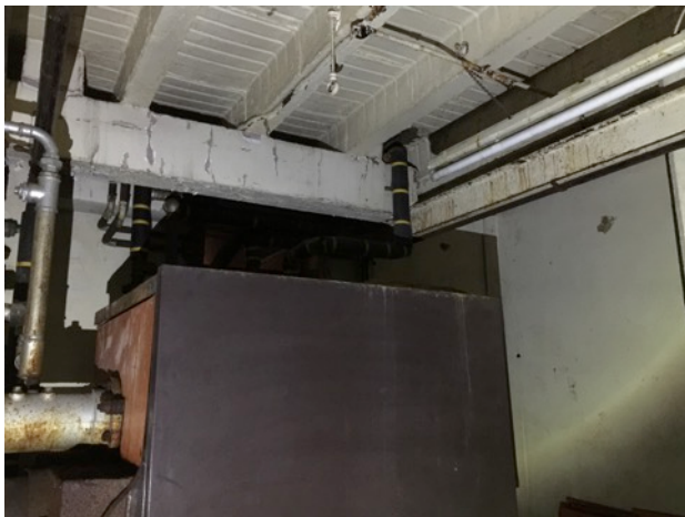
Photograph 16: One of the side rooms in Building 2.
