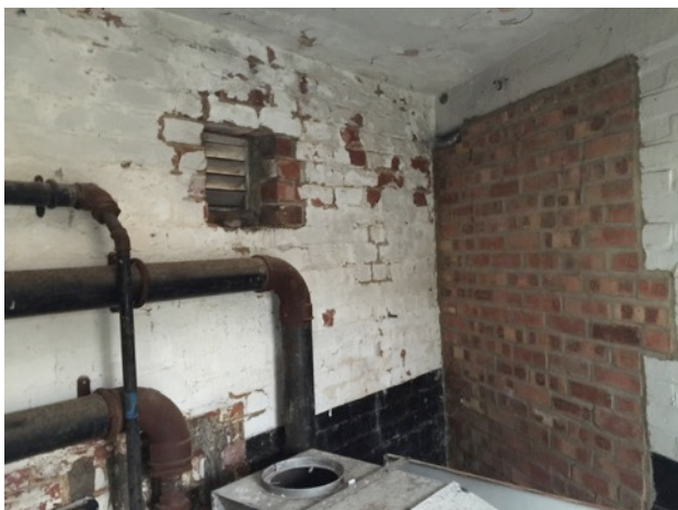
Photograph 11: One of the side rooms of Building 1.
