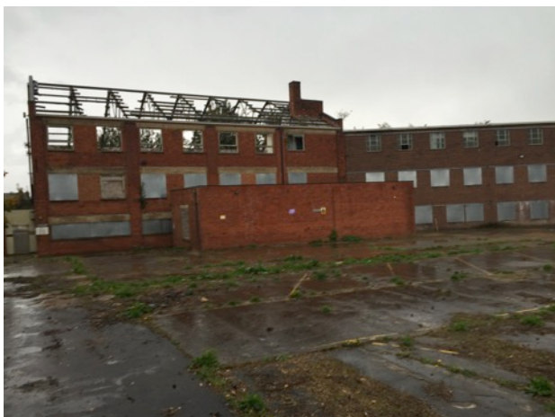
Photograph 17: View of lock up in front of Building 2.
