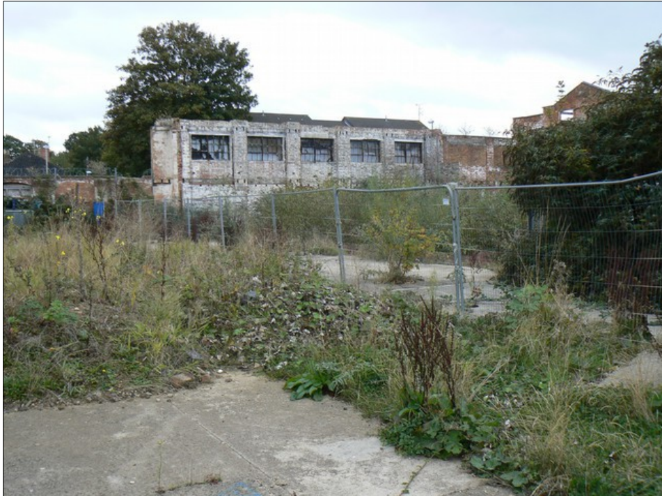
Plate 2: Demolished section of eastern range of buildings. View - SE
