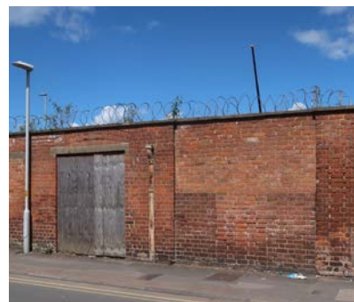
Existing heritage wall to be retained and made-good
