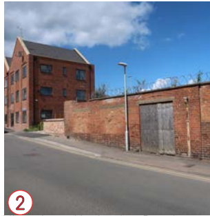
2 View from Hatherley Road, including access door.
