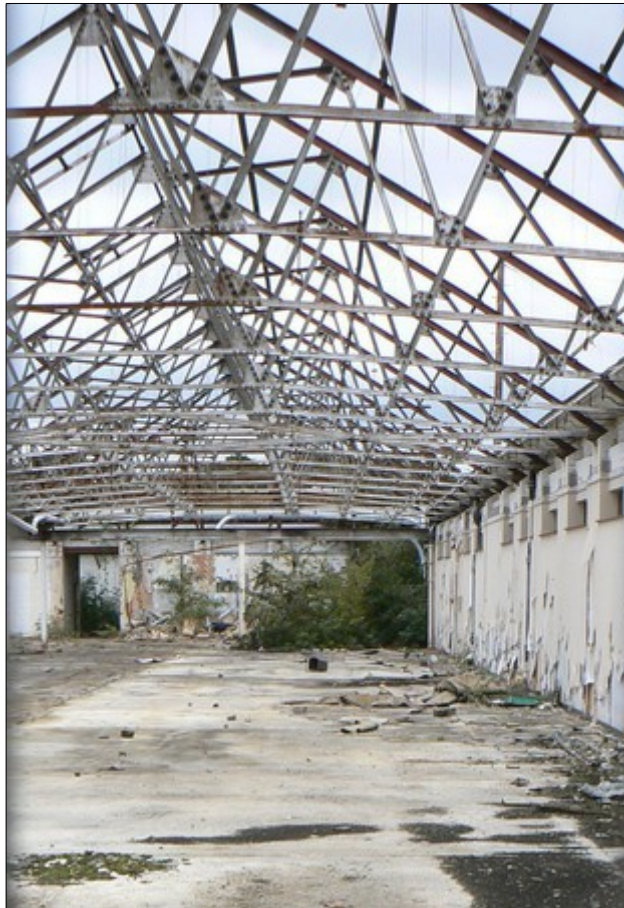
Plate 6: Interior of building in southern range. View - SE
