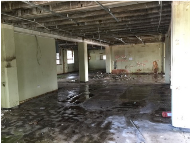
Photograph 15: Second floor interior of Building 2.
