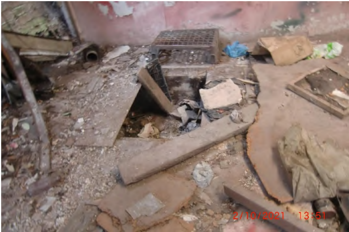
Inspection pit in mechanical workshop area, partially covered
